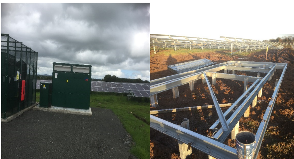
Figure 3 Rock fill with concrete plinth foundation and Piled alternative
