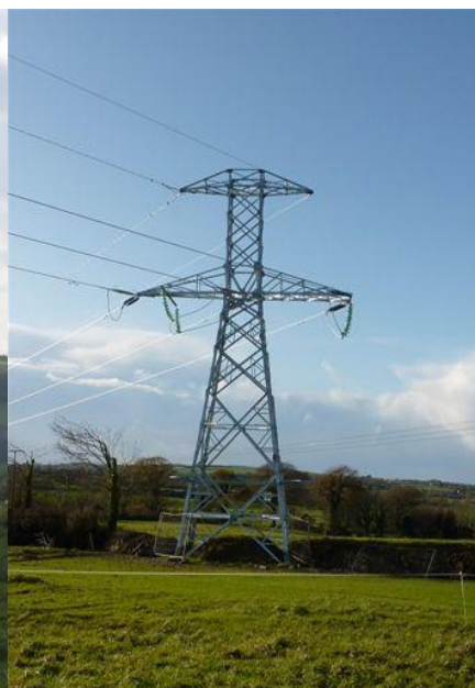
Figure 6 Typical steel angle structure
