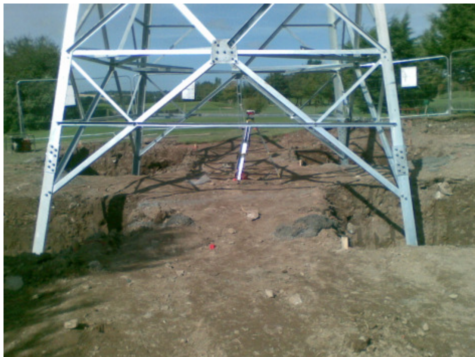
Figure 7: Photograph of steel tower base in open excavations
